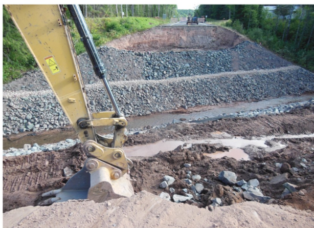
Hwy. 27 at Sandy Run Bridge Project looking south on August 22
