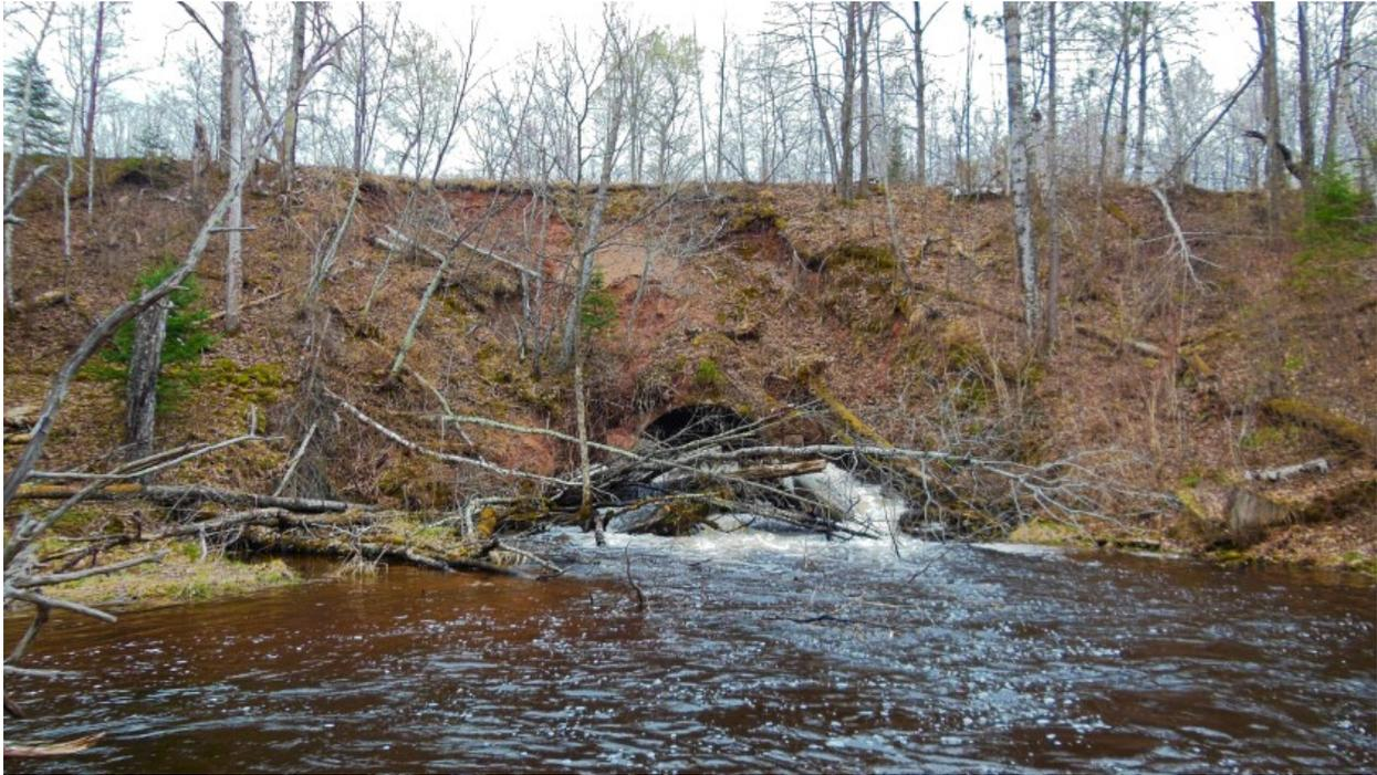
Before the recent project, a long-abandoned railroad crossing over Nebagamon Creek downstream from Lake Nebagamon had nearly plugged entirely, creating a damming effect that could have created a major washout, sending a torrent of water, sand and sediment downstream to the Brule River. The culvert and railroad grade were recently removed along the creek, creating a natural stream channel and removing the obstruction.
