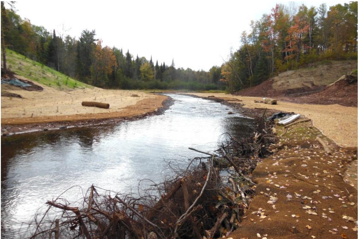
*With a blocked culvert and abandoned railroad crossing removed, Nebagamon Creek now flows freely and unobstructed from Lake Nebagamon to the Brule River. A \$770,000 project completed recently may have saved miles of fish spawning habitat along the creek and downstream river from a major washout.*
