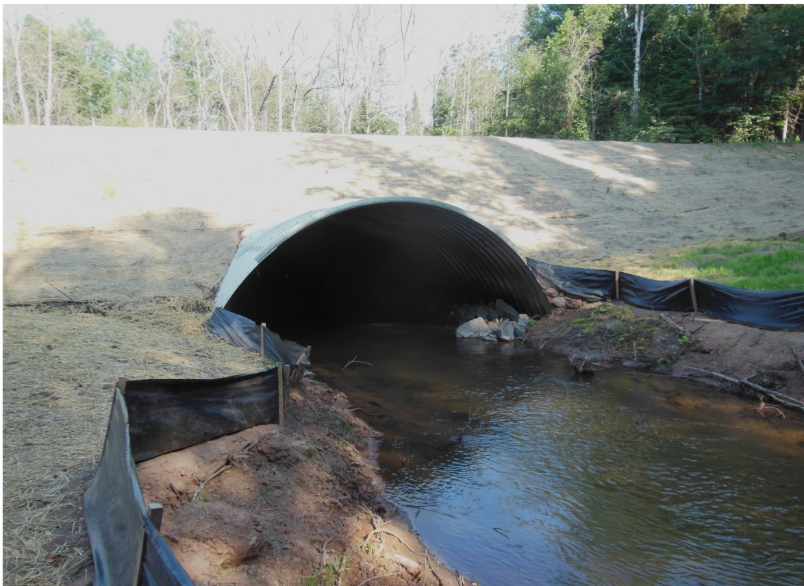
Newly installed culvert on the Little Brule at Ranger Road. Funded by NOAA, USFWS, Town of Brule, and TU.
