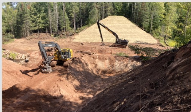
Site photo September 14 looking east (photo by Paul Piszczek)
