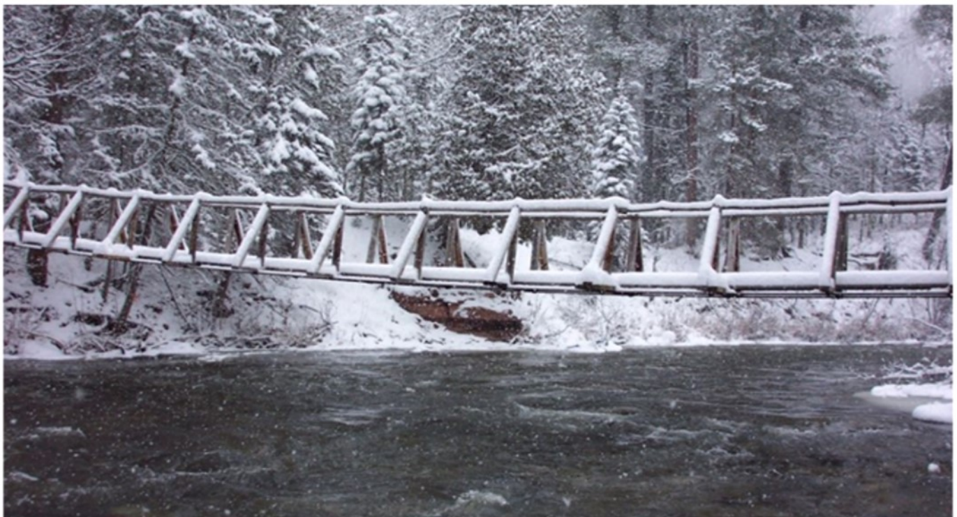
The swinging bridge on the Brule. - Photo taken by long-time Club member John Holter
