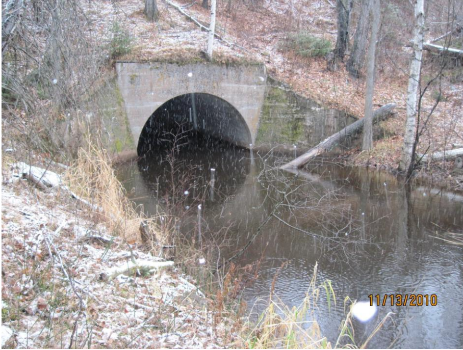
Figure 4. Culvert impounding water on upstream side of culvert.
