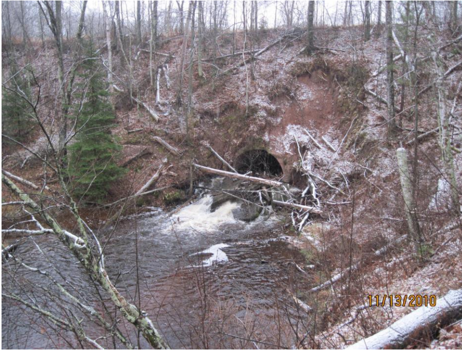
Figure 2. Wing-wall collapse at downstream side of culvert (Also note erosion of grade).
