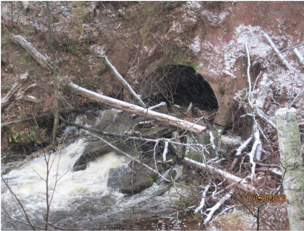
Figure 3. Close-up showing wing-walls entirely collapsed into stream.
